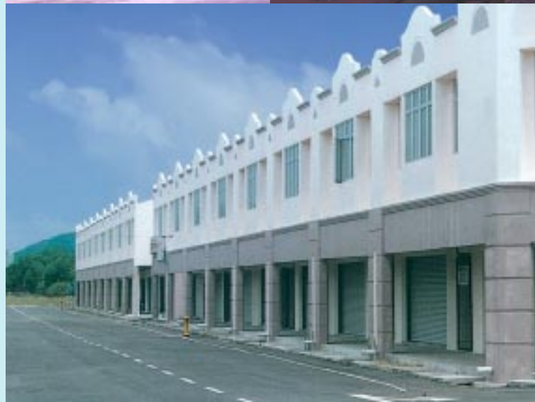
Completed shophots, Kerteh
