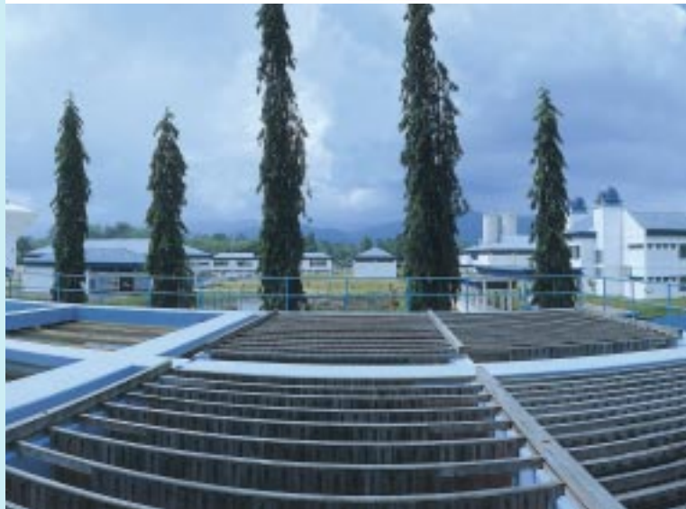
Water Treatment Plant, Terengganu
